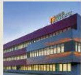
PRIMA INDUSTRIE HEADQUARTERS AND TECH CENTER Collegno (TO) - Italy
